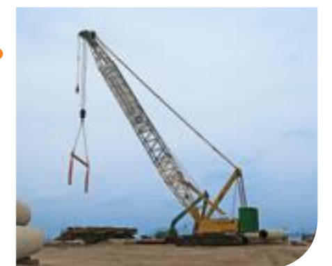
Submarine Pipeline - Butterworth to Penang
