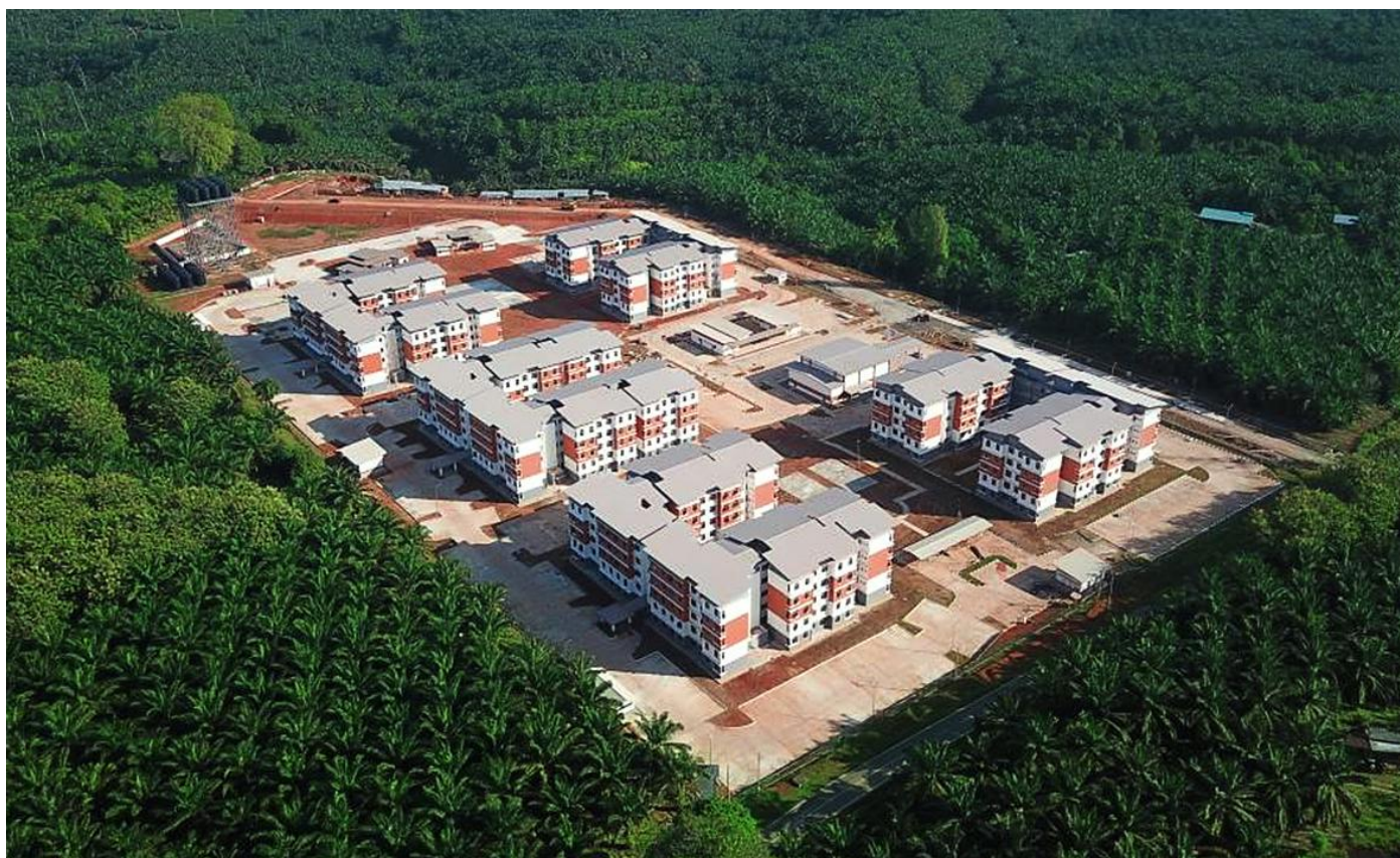
Tawau PPR, aerial view
