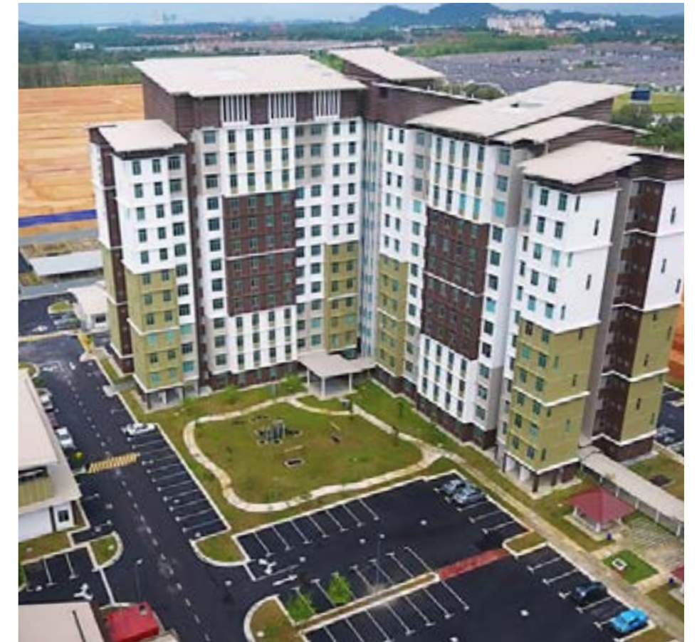
Ayer Panas PPR, Aerial View
